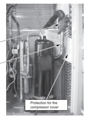
6. Place protective materials on the insulation lining of the compressor cover and on the sealing material on the compressor suction pipe to protect them from the torch flame, debraze the pipe, and replace the compressor.
