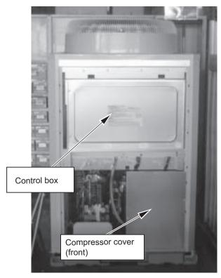
2. Remove the control box and the compressor cover (front).
